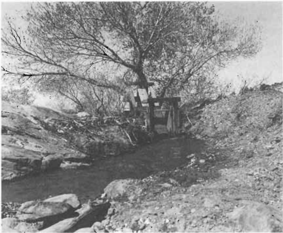
Diversion structure on Pleasant Creek dates from the 1920s. (Capitol Reef National Park Archives)
