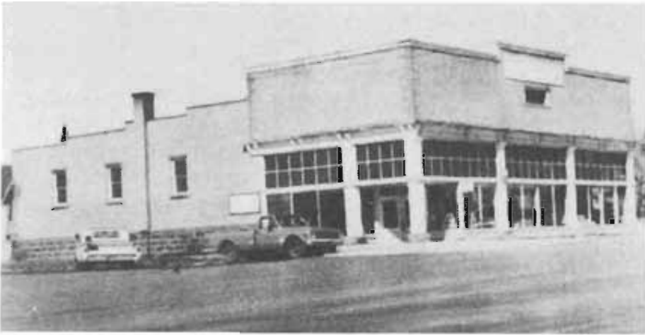
From 1912 to 1941 the Loa Co-op building housed county government. Now it is an inn. (Courtesy Barbara Ekker)
