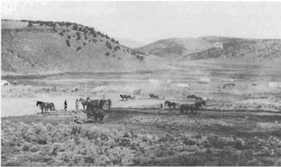
Construction crews and tent camp at Forsyth Reservoir site. (Courtesy Harold Brown)
