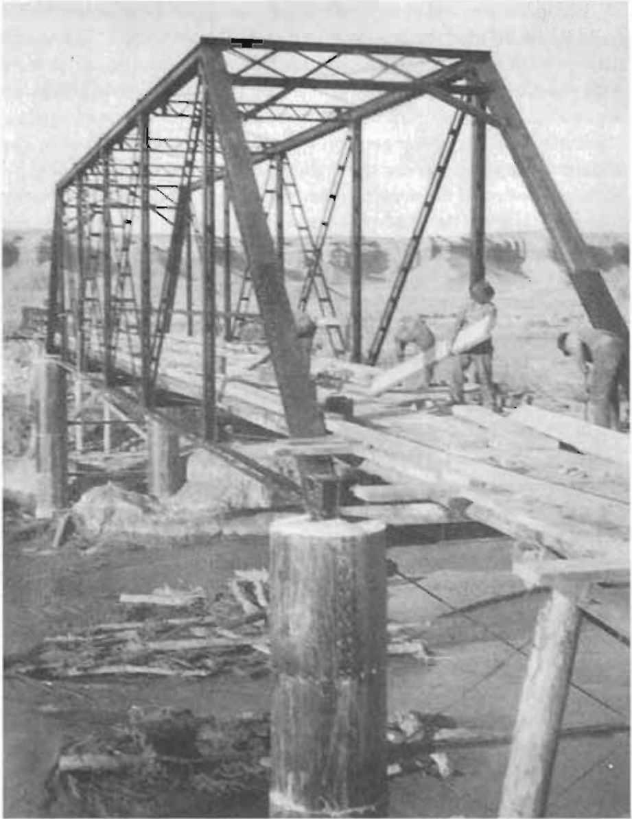
Construction of Hanksville bridge, c. 1921. State Road Commission photograph. (Utah State Historical Society)
